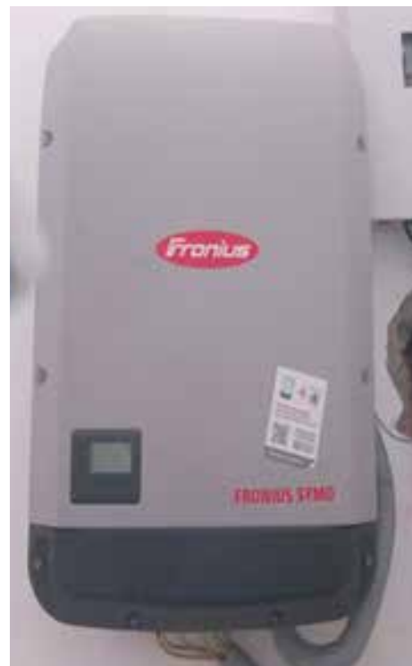
Picture 2: Inverter at Bansal's residence is Fronius Symo 20
