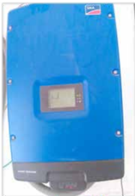
Picture 6: Inverter at Mr Kapoor's residence is SMA Sunny Tripower
